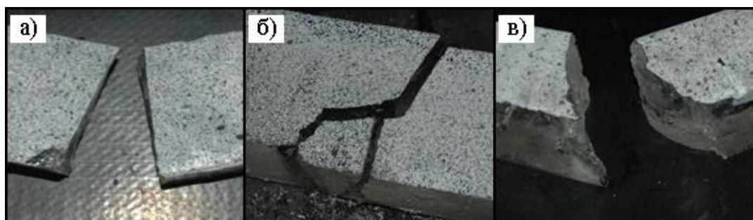
Figure 1.32 – Typical types of cracks: a) straight, b) zigzag, c) curve [2]
